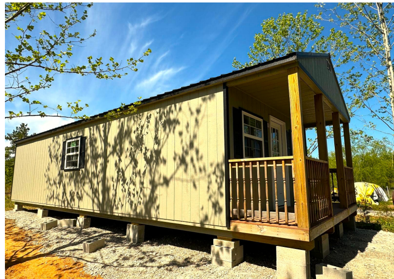
A Concrete or Compact Gravel Base is recommended to prevent settling as well as creating a moisture and pest free environment under your building
